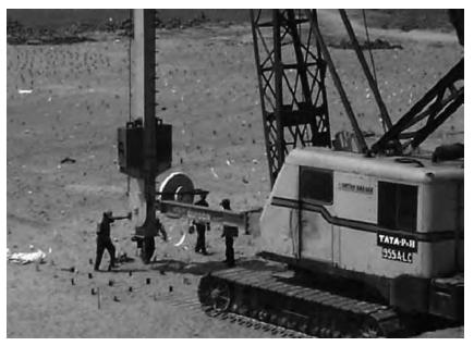
Fig. 5.2 Installation of Prefabricated Vertical Drains (PVDs)
