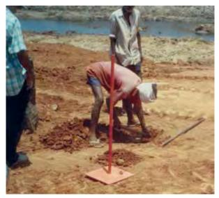
Fig. 6.5 Installation of Surface Settlement Marker (Settlement Platform)
