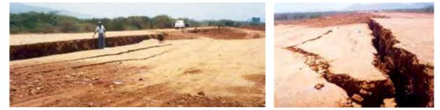
Fig. 6.1 Typical Failure of Embankment on Soft Sub-soil
